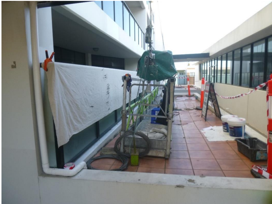
Figure 06. General view of the working platform/cradle.
