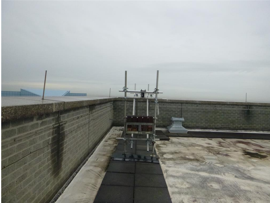
Figure 07. General view of roof mounted outriggers
