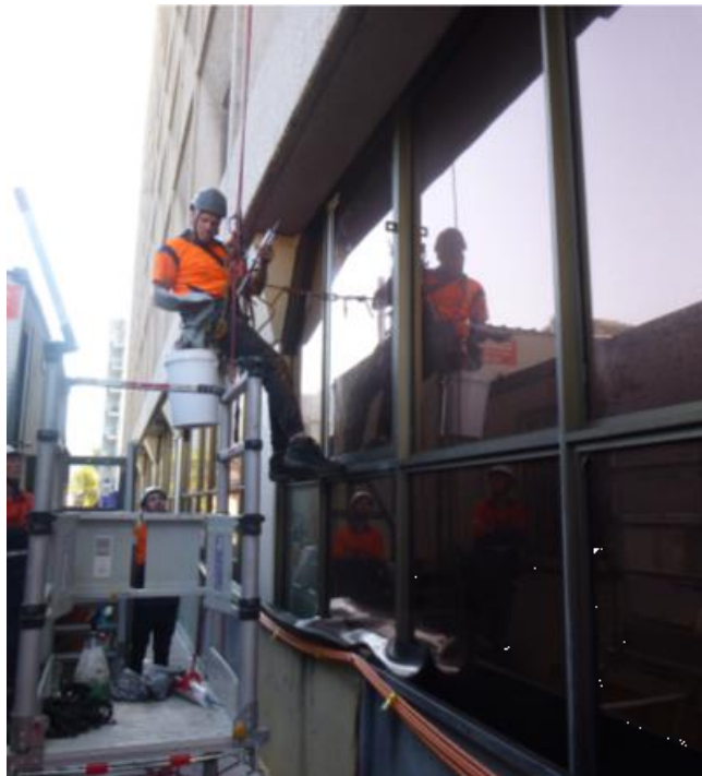
Figure 04. Façade resealing works in progress.
