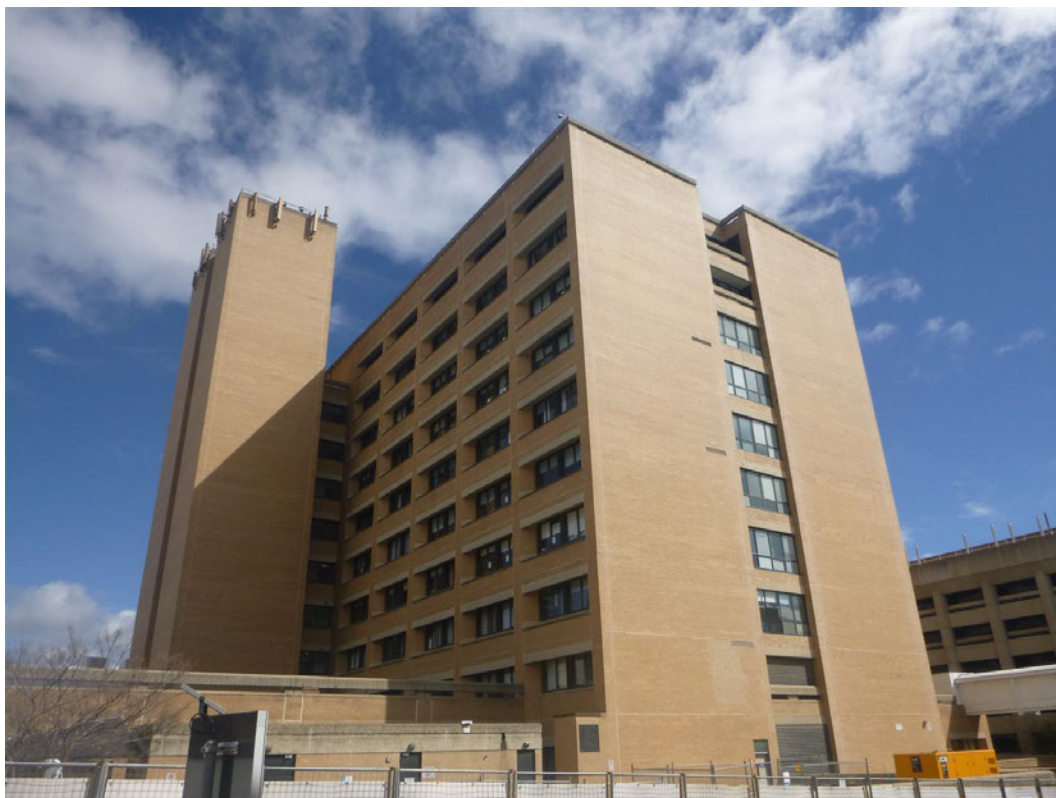
Figure 1: General view of Canberra Hospital's Building 1
